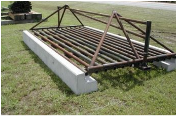
Buttress with steel rails on them.
