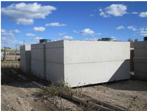
Combine cisterns for needed storage capacity.
